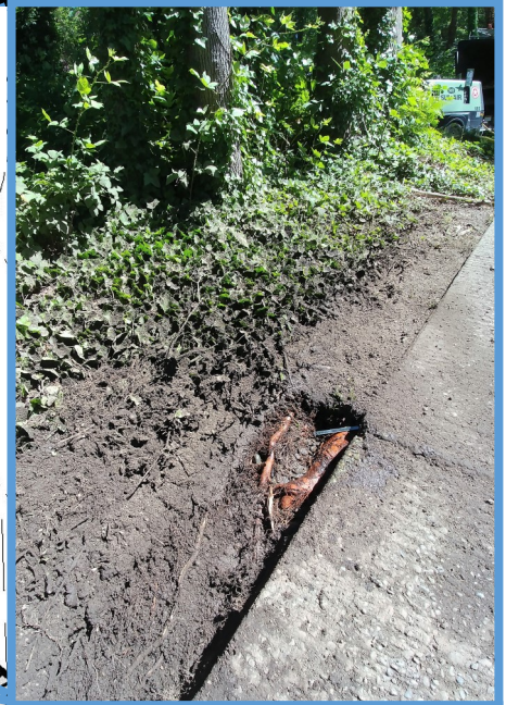
Photo A. Two three-foot long And four inch diameter maple roots at the top of the cut.
